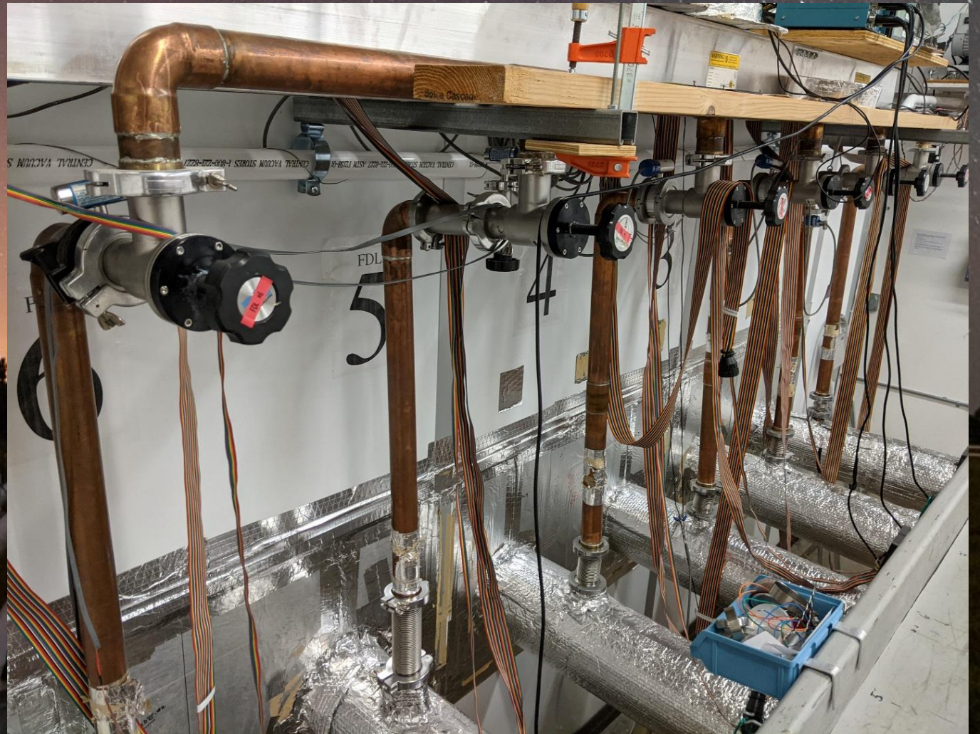
Connection of FDL to previous vacuum manifold
